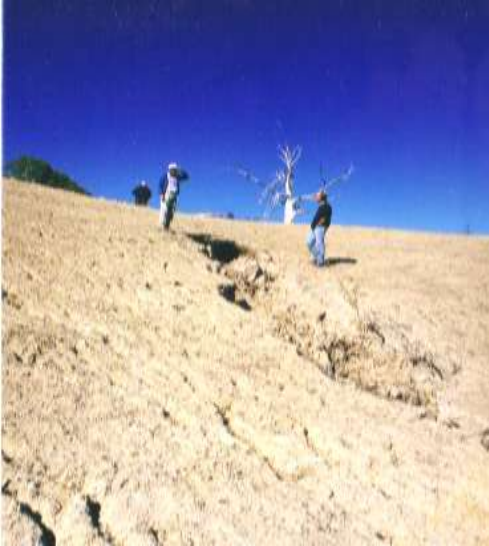
Figure 19: Rilling dam wall at Bimbimbie (source and date unknown).
