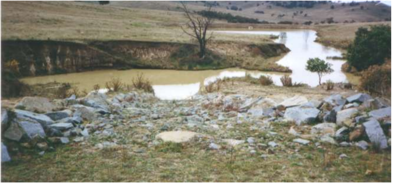
Figure 10: A rock flume controlling the entry of water at Woodborough (date and source unknown).
