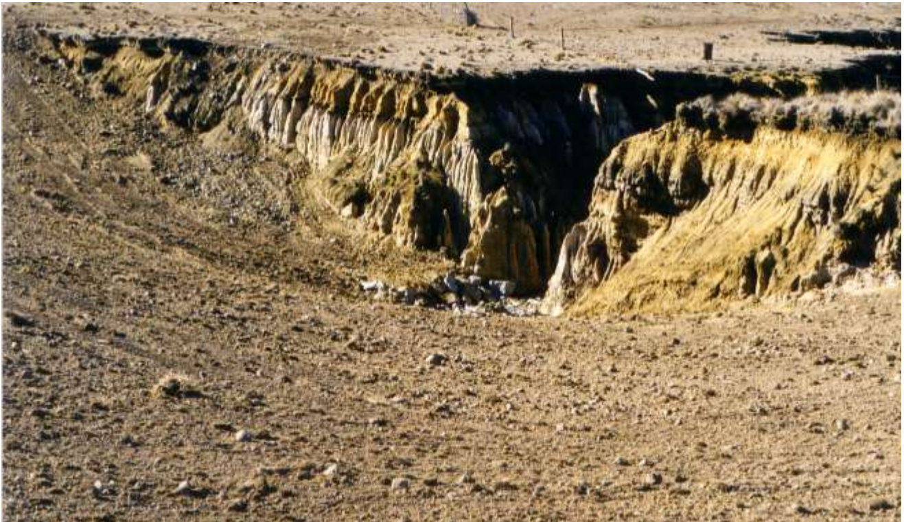
Figure 37a: Battered banks and a rock groyne at implementation, Woodborough (source and date unknown).
