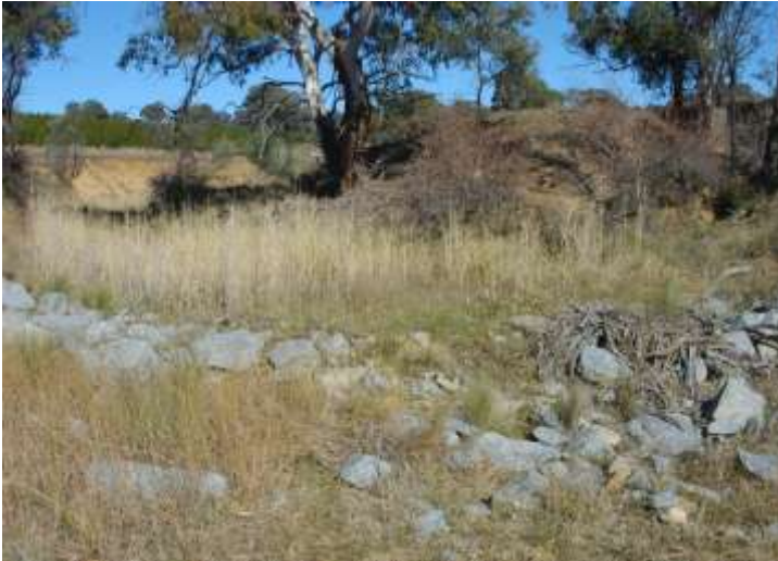
Figure 17a: A rock groyne trapping sediment in conjunction with Phragmites ( Phragmites australis ) at Airlie Park (courtesy Sally Anne Thompson 2007). This groyne has been highly successful, elevating the level of the bed with sediment, which has grassed up well. Although there has been some movement of rocks (as to be expected) there has been no significant impact on the structure by overland flow. It should be noted that the control of water by a sediment basin above, is essential in decreasing the
