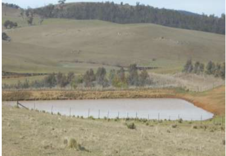
Figure 20: A sediment basin and revegetation at Wallendibby (courtesy Sally Anne Thompson 2007).
