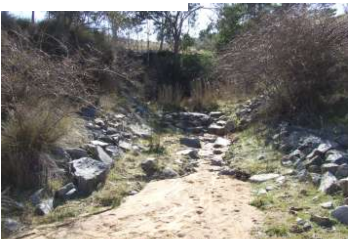
Figure 18: This figure demonstrates the finite capacity of rock groynes in relation to sediment input. This rock groyne at Corrowong, (which plays a final sediment retainment role before water is delivered to Corrowong Creek), is close to sediment capacity. Such a structure would benefit from the installation of a number of wire mesh weirs in the gully line above.
