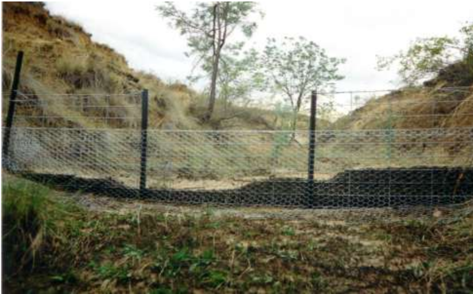
Figure 12: A wire mesh weir at Airlie Park shortly after construction (source and date unknown).
