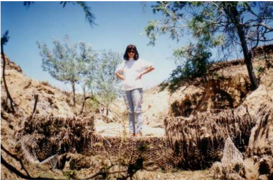
Figure13: Kerry Payten viewing the same wire mesh weir at capacity, immediately after an intense summer storm. Note the effect of raising the level of the gully floor by containing sediment (source and date unknown).
