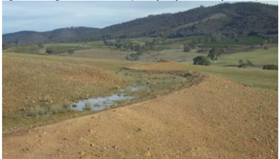
Figure 28: Diversion bank, Corrowong (figure courtesy Emma Platts 2007)
