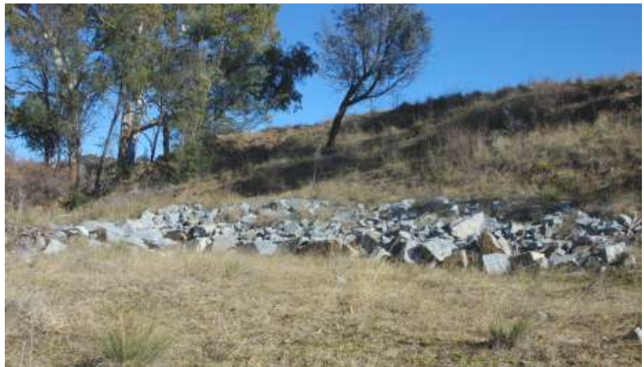
Figure 17b: Extension of the above rock groyne (a type of rock ‘sausage’) to armour the adjoining bank. This structure has also proved highly successful. Note grass establishment on the gully floor. The sidewalls were battered back by an excavator at the time of construction, affording grass species the ability to establish on a more stable grade.
